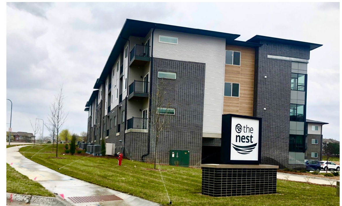
Figure 6: Employer-built housing in La Vista
